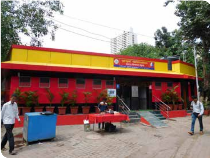
↑ CONSTRUCTION OF PUBLIC TOILETS COMPLEX AT MUMBAI
