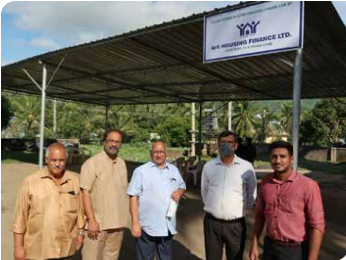
↑ GREEN INITIATIVE - SOLAR PANEL INSTALLATION AT KERALA
